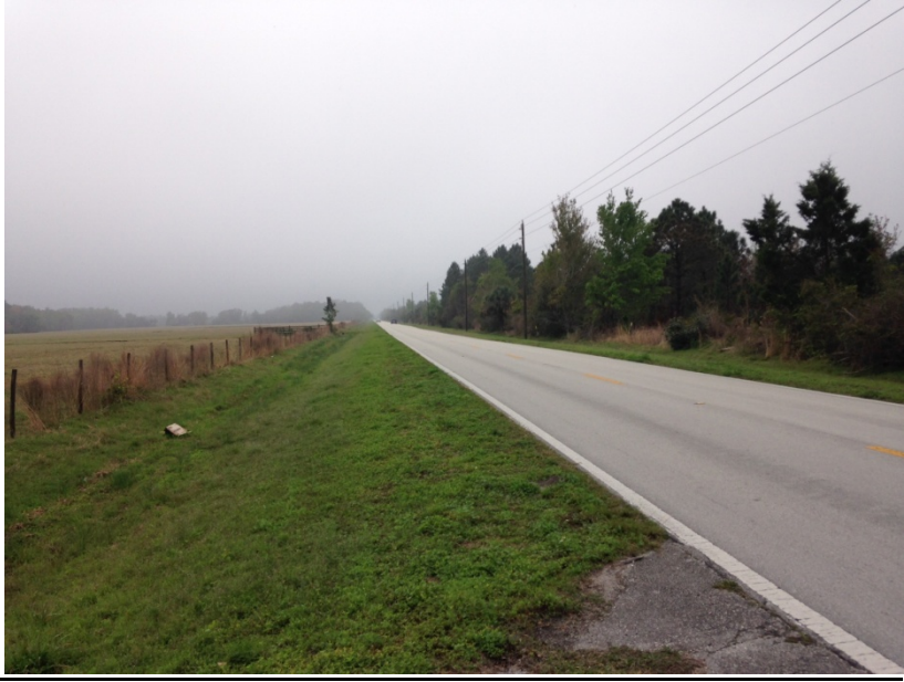
Street View – West
